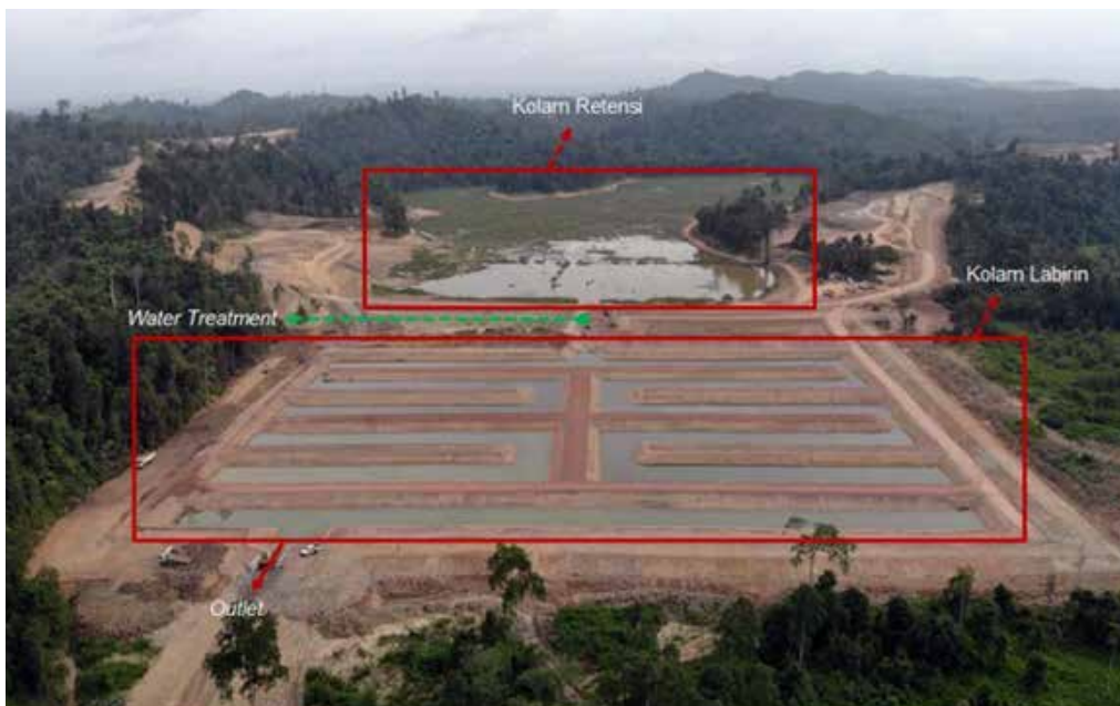
Drone Photo of Kemuning Pool
